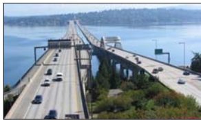
I-90 Floating Bridge
